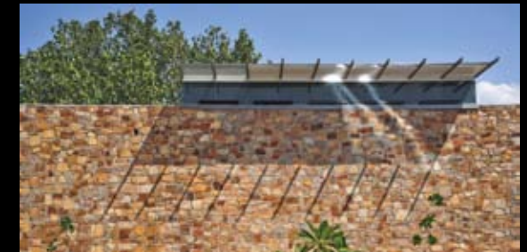
Stone, glass, steel and vinyl forms the basic palette for the architecture
